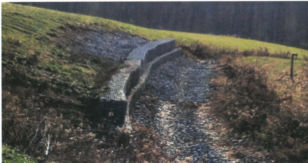
PHOTO 1: ADDITIONAL EROSION REPAIR - GABION CAGE EXTENSION
