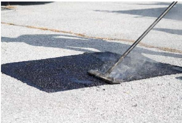
**What is it?** Hot Pour Mastics (HPM) is a technique that can be used year-round as a one-time application to fill large cracks and small potholes in concrete and asphalt pavements when surface temperatures are 40 degrees Fahrenheit and rising. It combines the flexibility and adhesion of rubberized asphalt sealants with the strength and load bearing capabilities of engineered aggregates.
