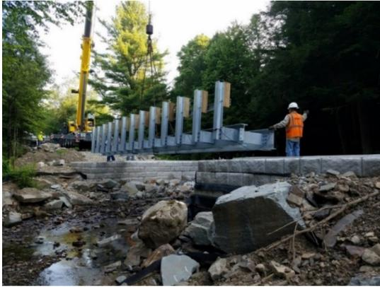
**What is it?** Geosynthetic Reinforced Soil-Integrated Bridge Systems (GRS-IBS) is an Accelerated Bridge Construction method which uses alternating layers of geotextile material combined with crushed and graded stone and concrete facing blocks to construct the bridge abutments. The IBS is created when the superstructure (typically beams and deck) is placed on top of the GRS abutments to create the bridge.
