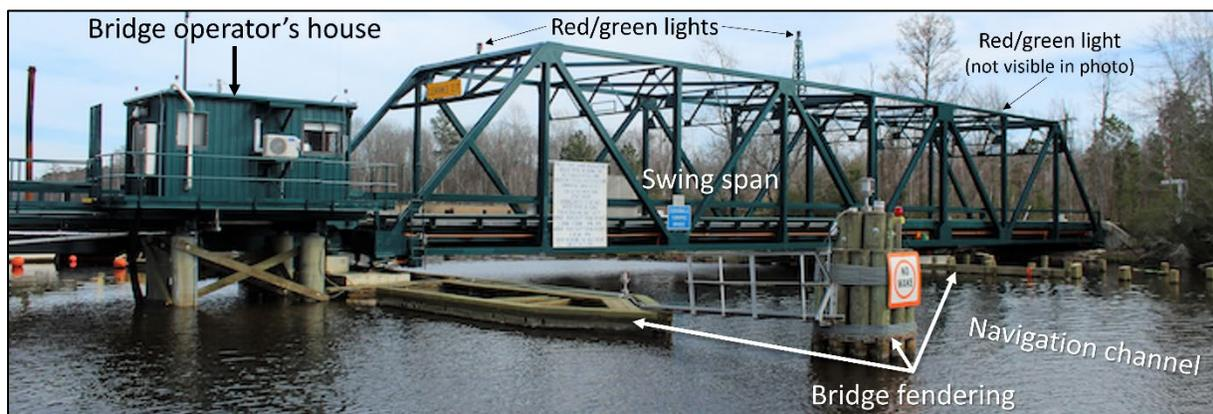
**Figure 3.** Centerville Turnpike Bridge in the closed position. (Source: City of Chesapeake)
