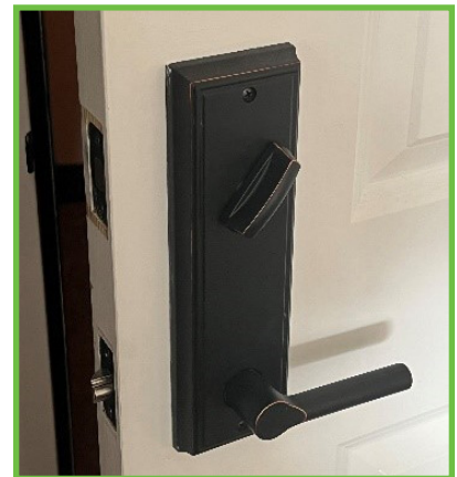
Rotating lever retracts latch and deadbolt.
