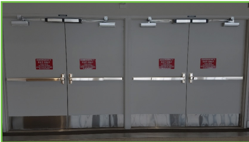
Delayed egress door with electromagnetic locks (mag locks) and door closers.
