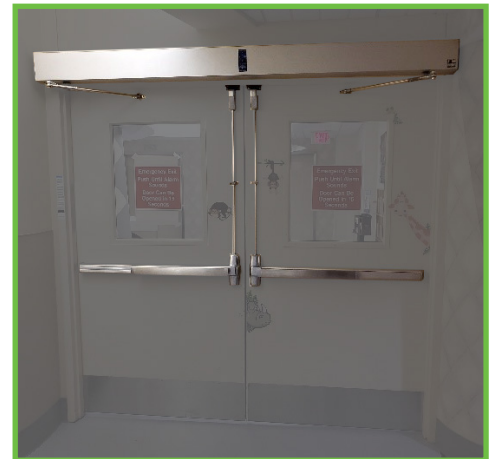
Delayed egress door with power door operators.
