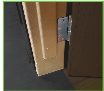
Door frame with terminated stop.
