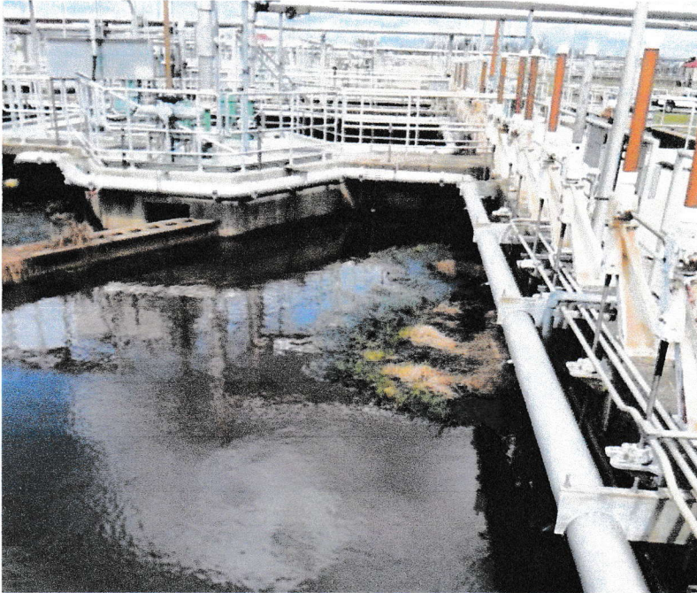
Solid's accumulation in the one of the reactors 3/26/22
