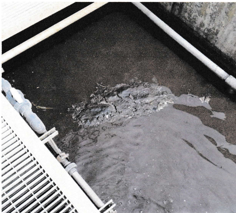
Floating solids in one of the reactors 3/26/22
