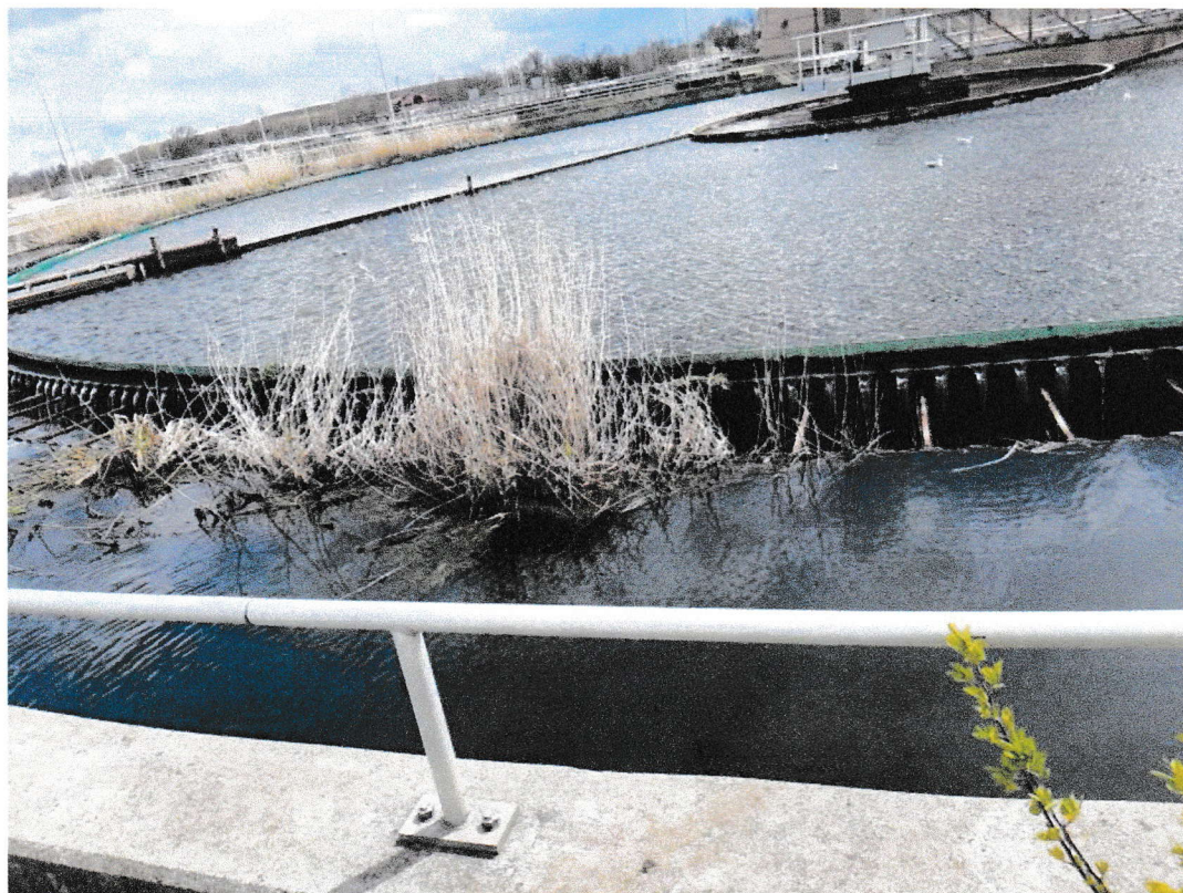
3/26/22 Secondary clarifier- vegetation and solids clogging the system and short-circuiting of the weirs.
