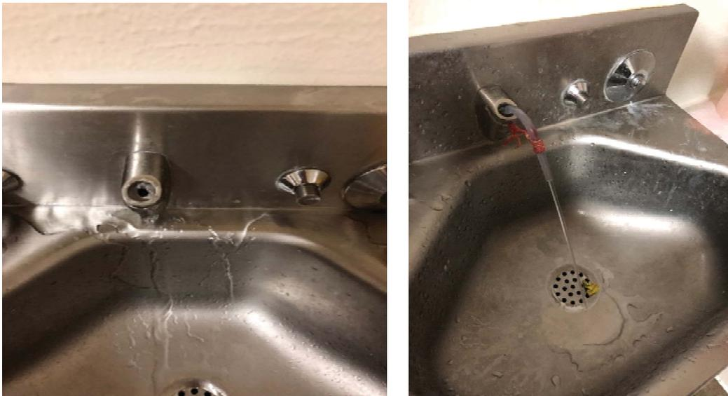
Figure 5. Leaking faucet without plastic straw (left) and faucet with plastic straw (right) observed by OIG at Baker on July 30, 2019.
