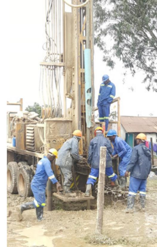
Through its WASH program, MSF has rehabilitated 70 existing boreholes providing safe and sufficient water to communities and institutions like churches, clinics and schools across Harare since 2015. These boreholes were rehabilitated using a unique borehole diagnostic tool kit, mounted in a self-contained vehicle.
